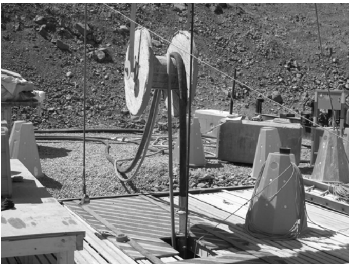
Figure 12. Cable reel over which the pump and air hoses pass.
