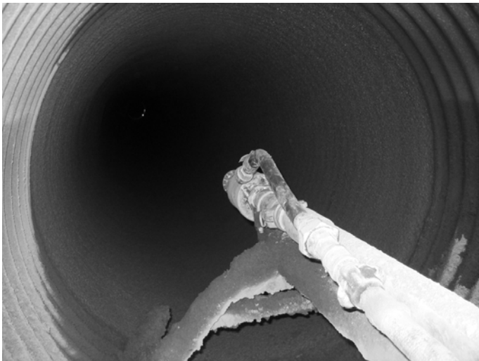
Figure 7. Robotically applied centrifugal sprayed concrete lining horizontal metal culvert.
