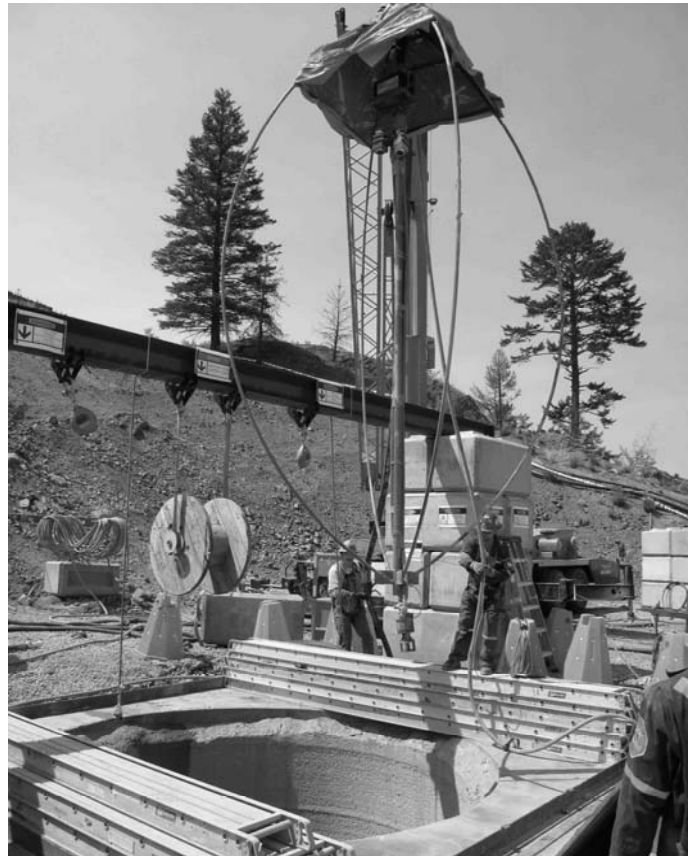
Figure 8. Top of raise bore shaft prior to centrifugal sprayed concrete lining.
