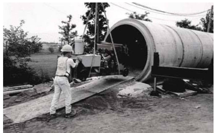
Figure 1. Robotic lining of pipe with conventional wet-mix shotcrete.
