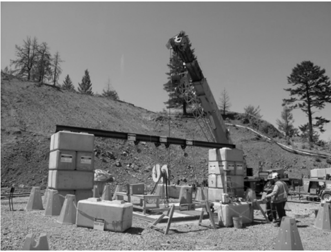
Figure 10. General rigging set-up for CSC lining of raise bore shaft.
